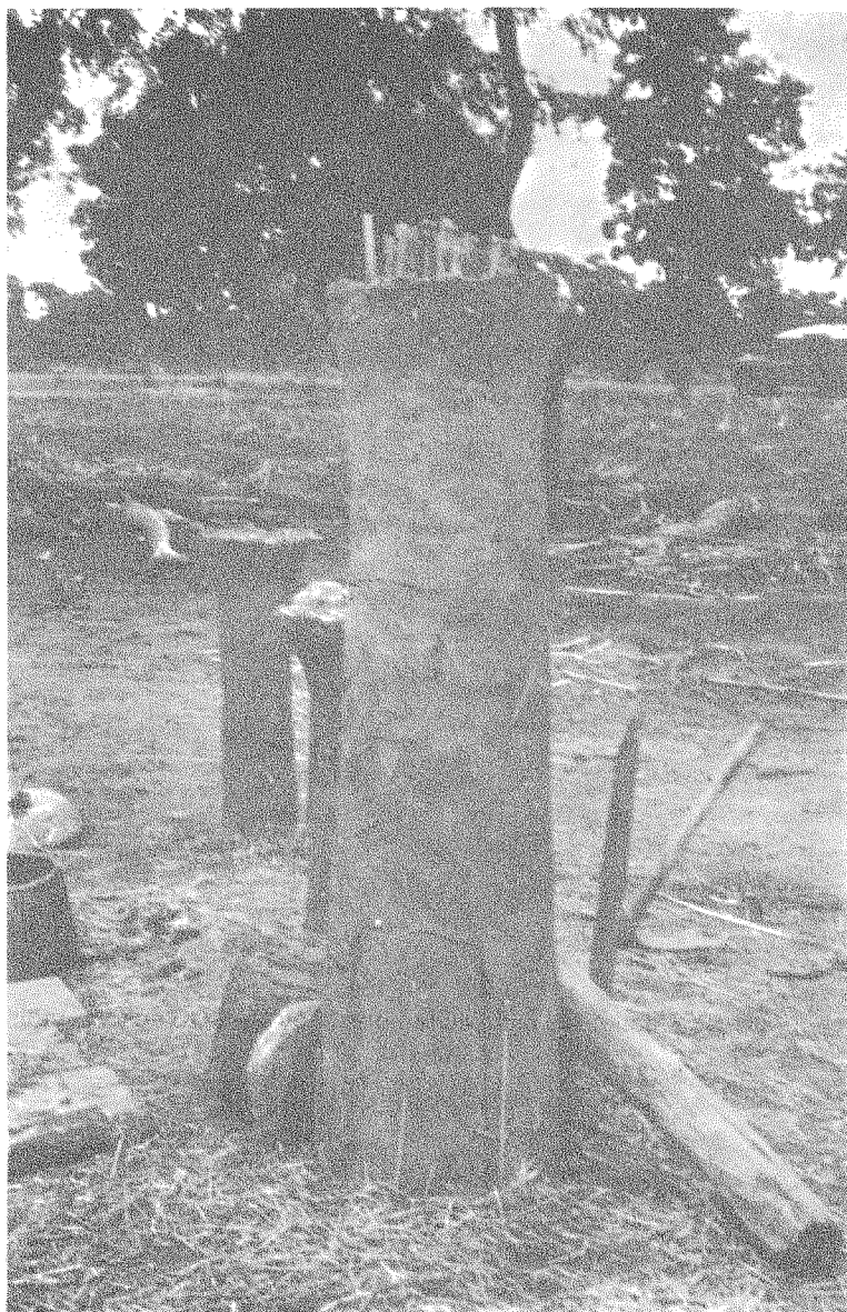
Plate VIII Tiza; shaft after one day's work. Note protective sticks in position.
