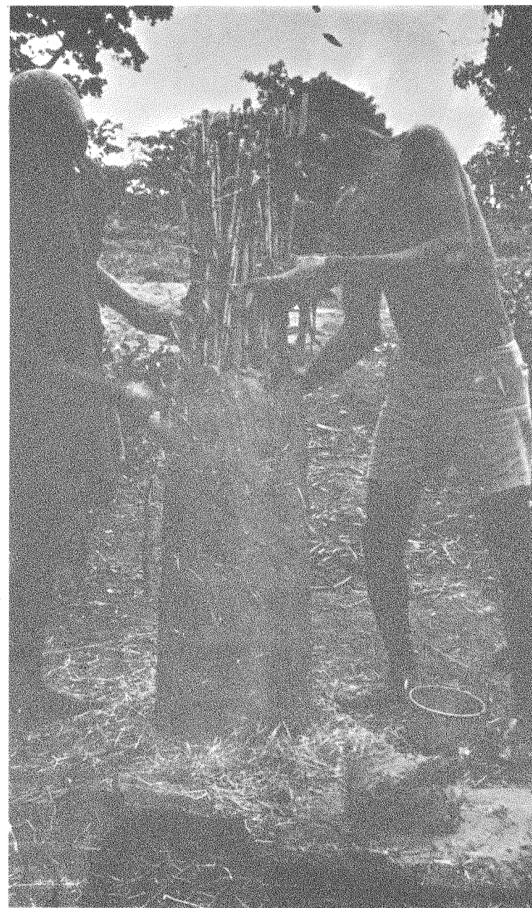
Plate VI Tiza; shaft being moulded around a core of guinea-corn stalks.
