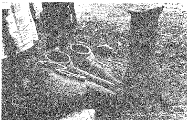
Plate IV Furnace at Chiana; note upright shaft, two low pairs of bellows. Height of shaft 122cm (57").
