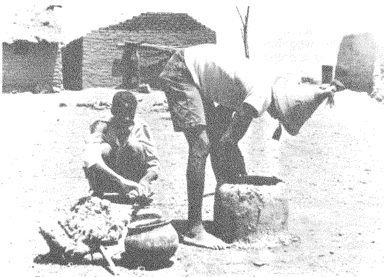
Plate XI Jefisi; shaft being built up with slabs of clay.
