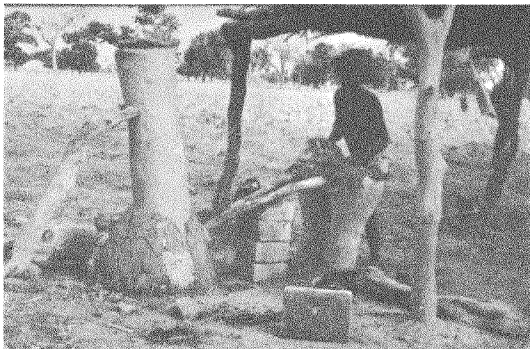
Plate III Furnace at Tiza; height of shaft 155cm (73").
