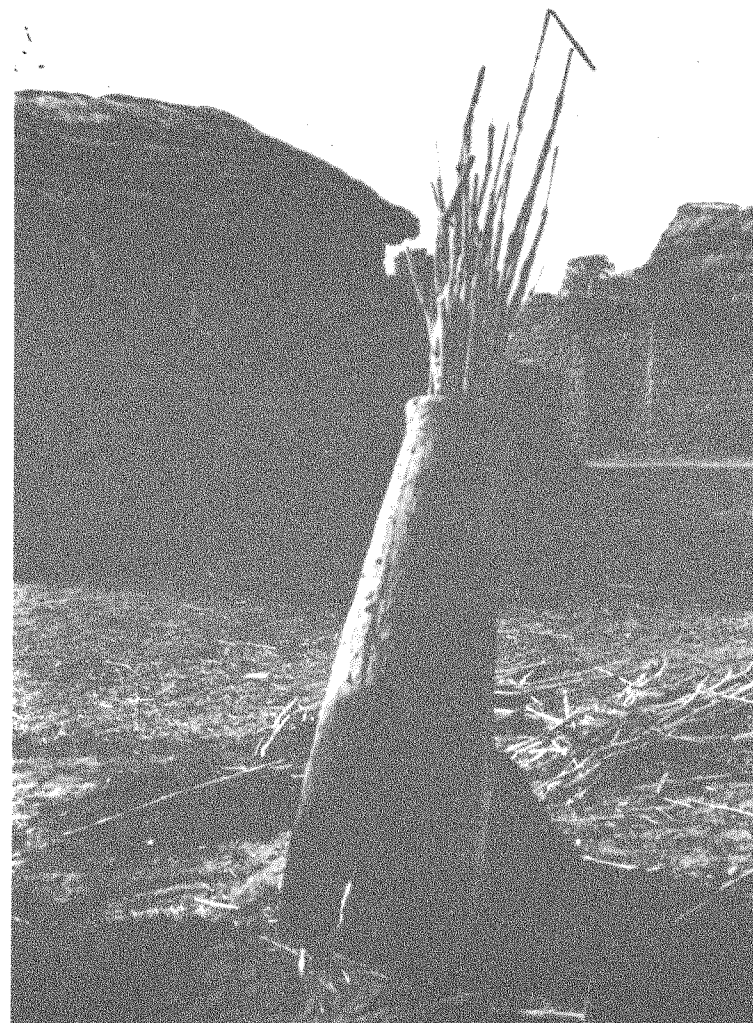
Plate XVI Jefisi; guinea-corn stalks lit in the shaft at start of smelt.
