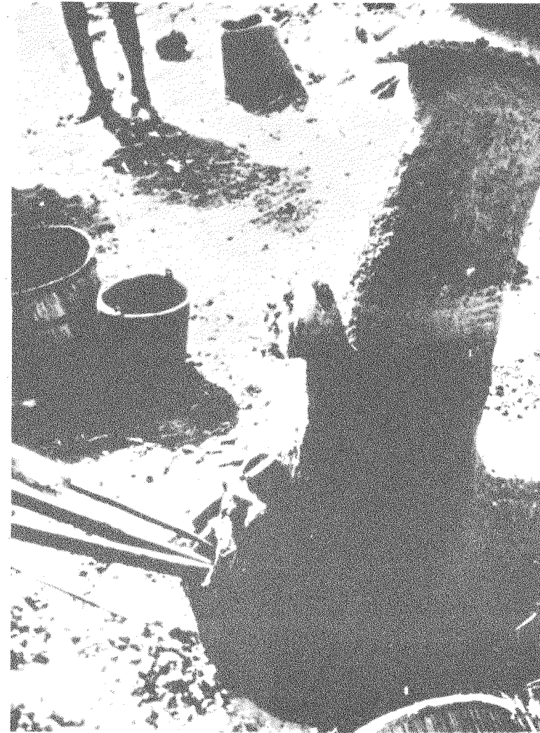
Plate II Furnace at Lawra; note remains of sacrifice on 'navel' and chicken roasting above tuyere. Height of shaft 135cm (63").
